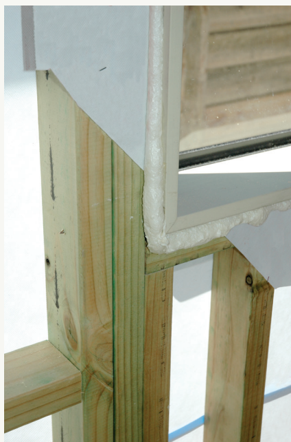
Continuous air seal before trimming.
